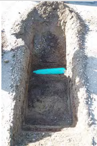
Figure 10: Exposed service in MT107. Area F.
