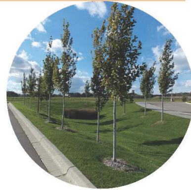
Dry Swales & Enhanced Grass Swales
