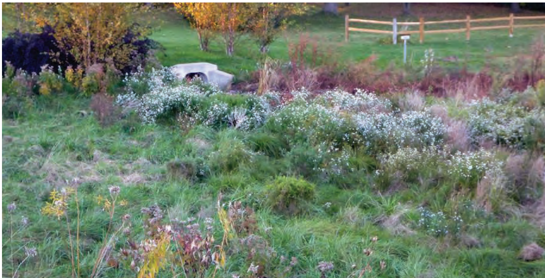
Figure 39. Native, deep-rooted vegetation in a stormwater detention basin
