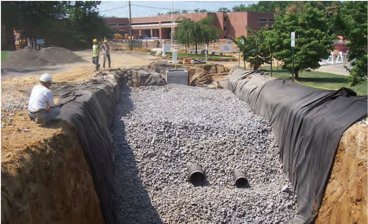
Figure 33: Construction of gravel infiltration gallery
