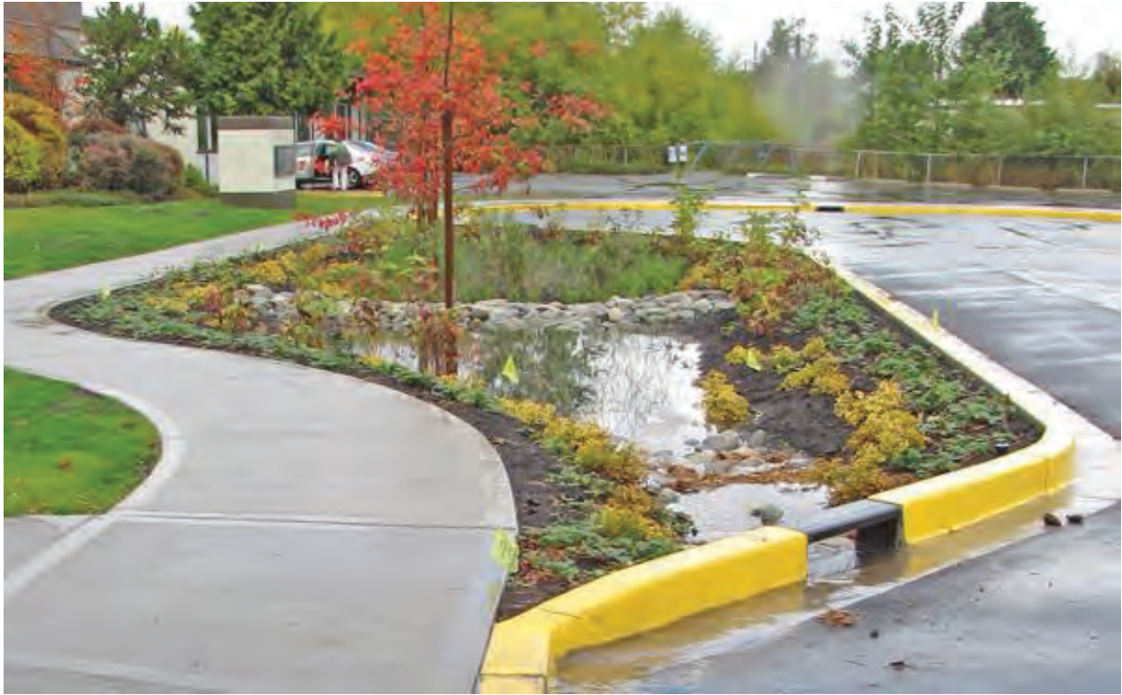
Figure 35. Rain garden with curb cut inlet for roadway runoff
