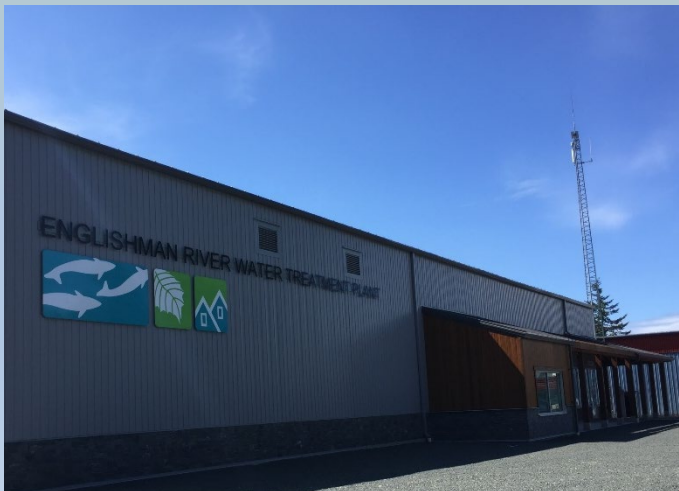
ERWS Water Treatment Plant
