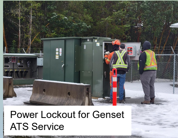
Generator Automatic Transfer Switch
