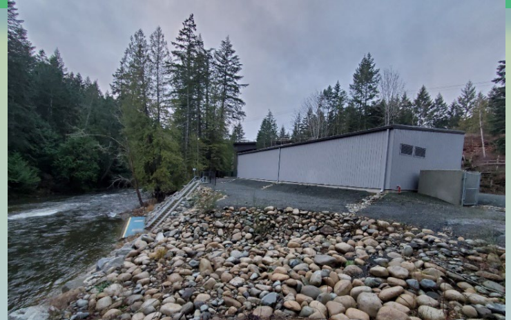
River Intake & Raw Water Pump Station
