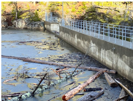
Arrowsmith Dam – Debris accumulation
