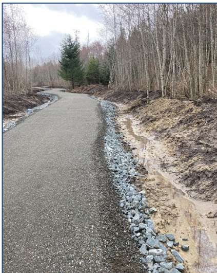
New trail with berms helps to eliminate trampling off trail.
