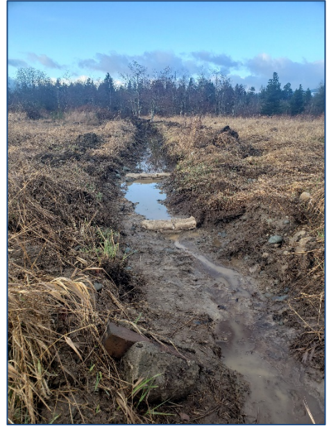
Hirst Avenue drainage (above)
