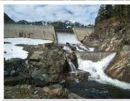
ARROWSMITH LAKE DAM ELV = 828.50m
